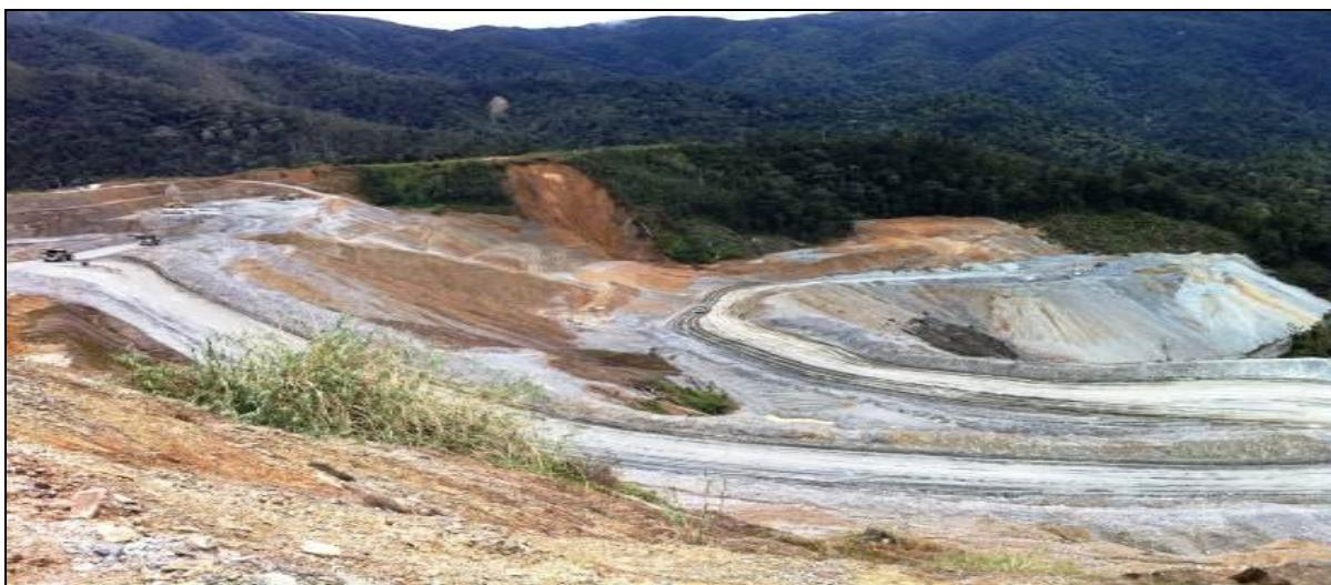
**Figure 19:** Construction of engineered bottom-up waste rock dump at Nosave
