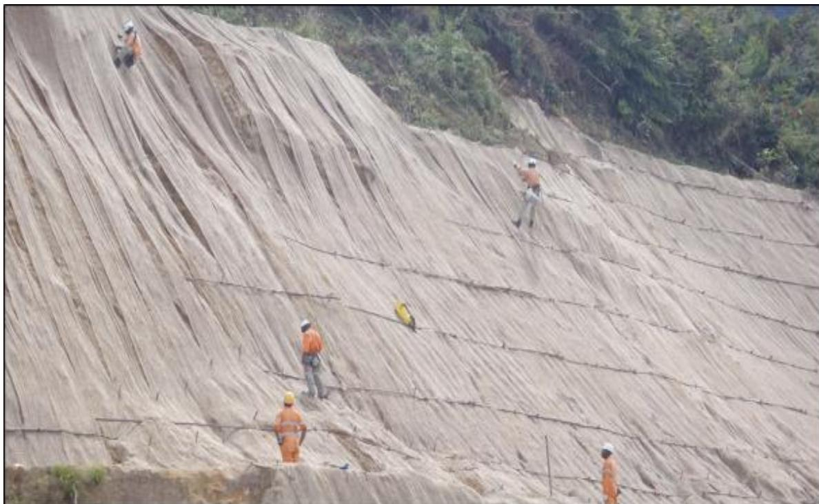
**Figure 22:** Environment Team stabilizing a steep exposed slope.
